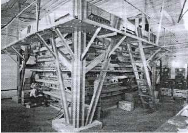
Figure 2. The ionization sampling calorimeter of Babayan, Grigorov, Shestoperov and Sobilyakov used in conjunction with nuclear emulsions.
