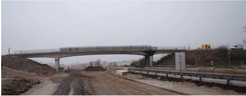
Figure 6: S101 Bridge before demolition.
