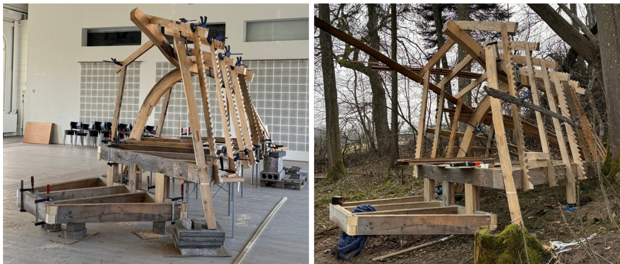
Figure 5: ReShelter construction phases.
