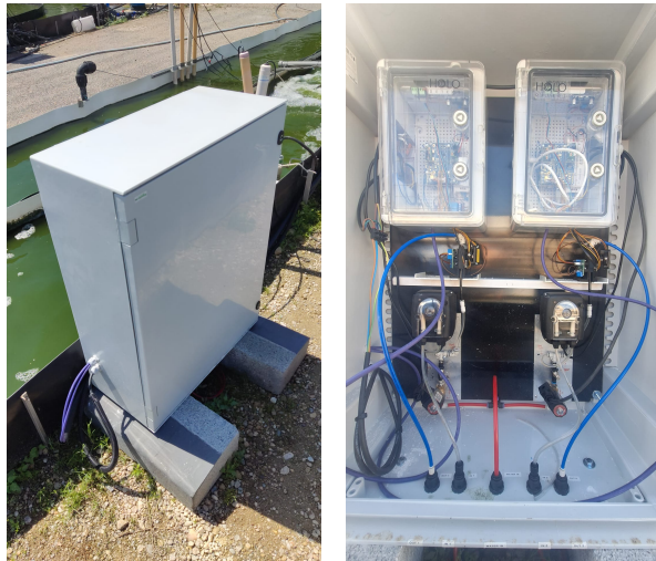
(a) External view of the sensing system installed next to the raceway reactor. (b) Internal view of the sensing system showing pumps, electronics, and flow-through measurement setup.
