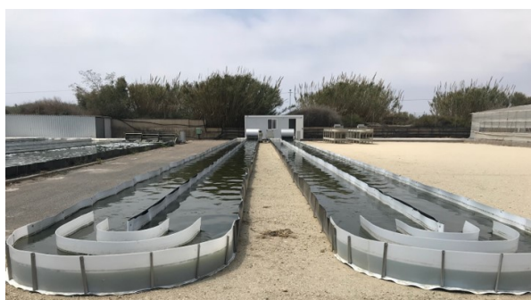
Figure 1: Outdoor 80 m 2 raceway photobioreactors (RW5 left and RW6 right) at the IFAPA experimental facility used in this study.
