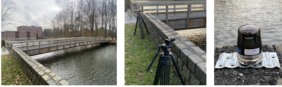
Figure 6: Overview of the data acquisition setup. From left to right: bridge overview, stereo vision configuration, and accelerometer installation on the bridge.
