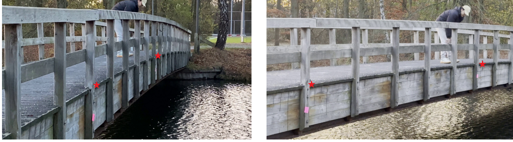
Figure A.15: Overview of the smartphone-based stereo sequence (Data-4). The two images show the first frames from the left (camera 1) and right (camera 2) views. The sticky notes placed on the bridge are used solely to expedite setup by facilitating localization of the monitored region within the FoV, rather than for tracking. The red stars indicate the locations of the accelerometers.
