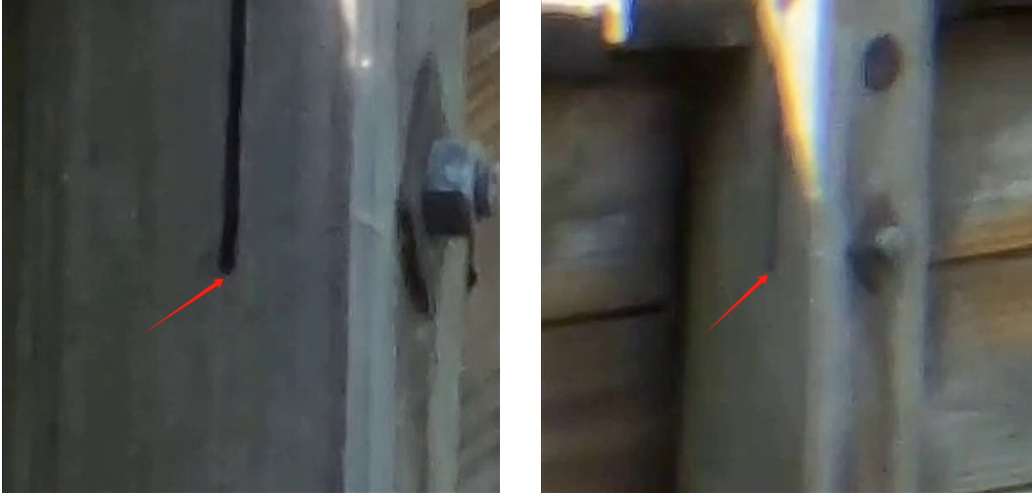
Figure 8: The first ROIs at the 1/4-span location of the bridge in Video-1 (left) and Video-2 (right) from Data-2. The red arrow indicates the tracked point.
