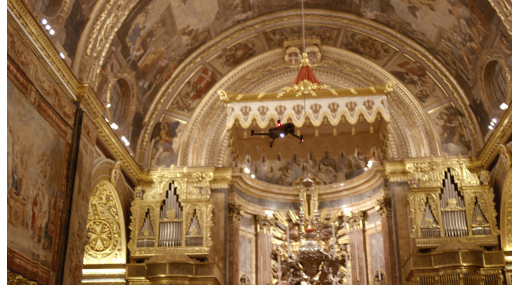
(b) Drone photography of ceiling
