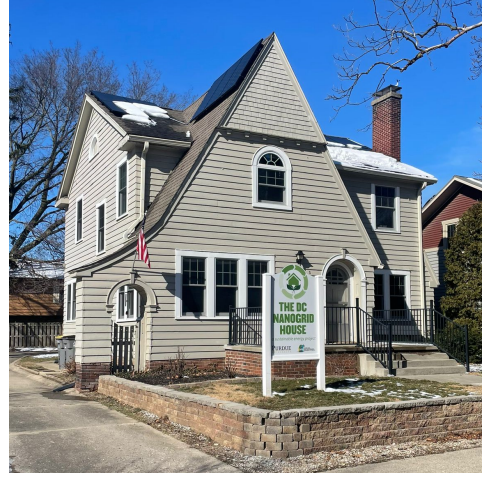
Figure 3: The test house is a 208 m 2 , 1920s-era detached house with all-electric appliances in West Lafayette, Indiana.
