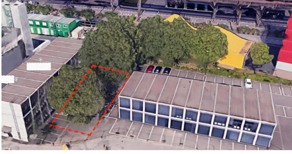
Figure 3: Picture captured from Google Earth. The area highlighted in red is where the experimental test is conducted
