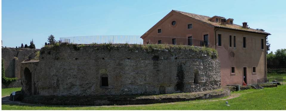
Fig. 2. The current state of the Maxentius Mausoleum. Only the Krypta still remains. The front porch is partly missing and has partly been used to build a farmhouse.
