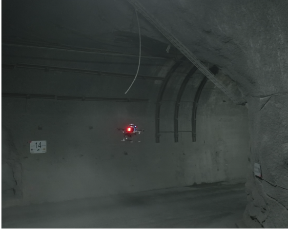
(b) Inspection mission in the Somport Tunnel , where poor light conditions, dust and changing winds are encountered.
