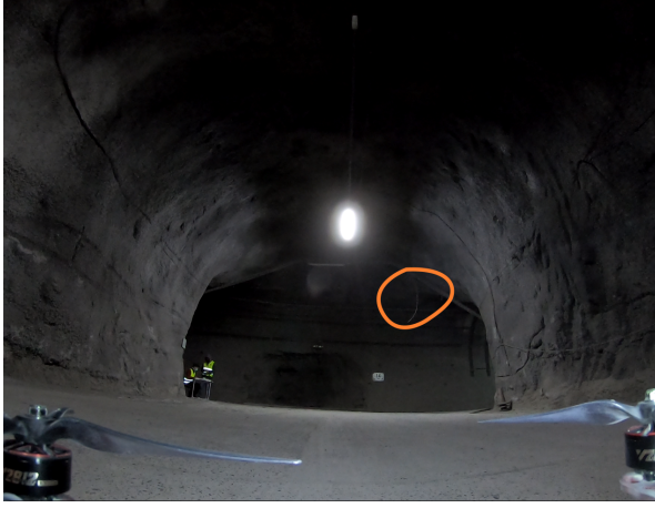
(a) View at takeoff point. Notice the thin wire at right hanging from the ceiling (circled in orange). The slope of the gallery until the intersection with the main tunnel can also be observed.
