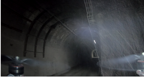
(b) Frame captured while entering the main tunnel. The sudden wind blows dust towards the camera. Dark regions of the tunnel can be observed after turning around the corner.
