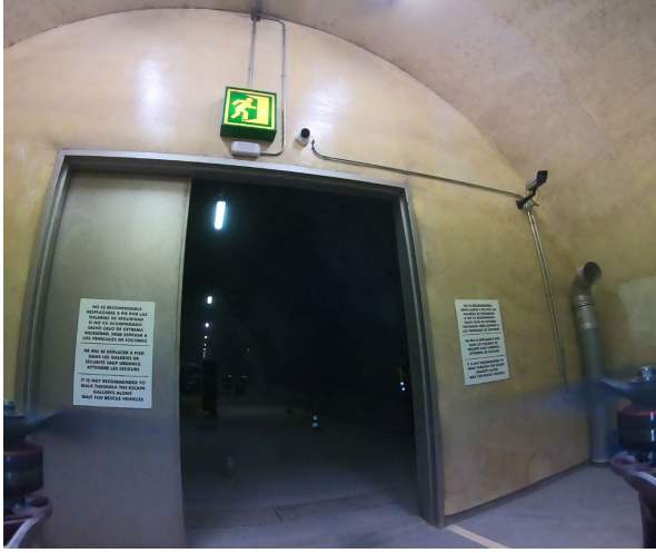
(b) Room inspection has been performed and return is started. Note the significant lighting differences inside and outside the room.
