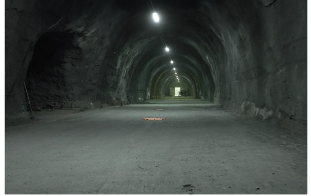
(a) Somport lateral gallery 14. The target room of the first mission is at the background. The orange circle at the ground is the second inspection starting point.
