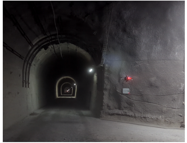
(b) Intersection between the main tunnel and gallery 14. The main tunnel leads to Spain in the direction in which the image was taken. Strong variable winds blow coming from Spain to France. Both the wind and the UAV flight lift dust that would severely affect a visual-based perception system. Additionally, the main tunnel is poorly illuminated in several regions.
