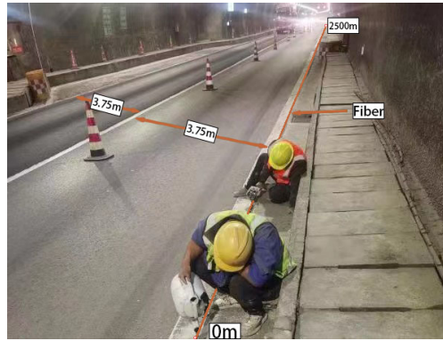
Fig. 13: Overhead view of the Jiurui Tunnel, and the optical fiber with a length of 2500m is laid on one side of the road.
