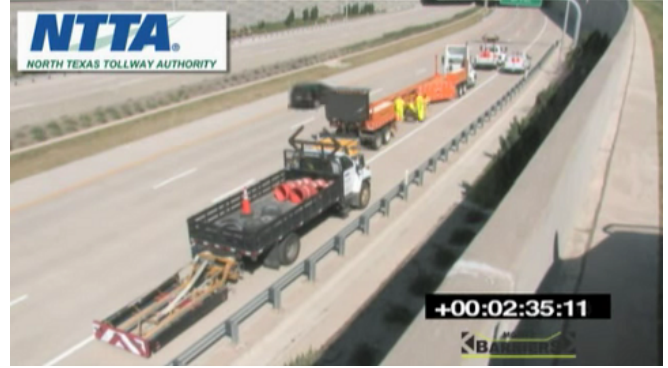
Fig. 1. Attenuator Truck Setup During Highway Work
