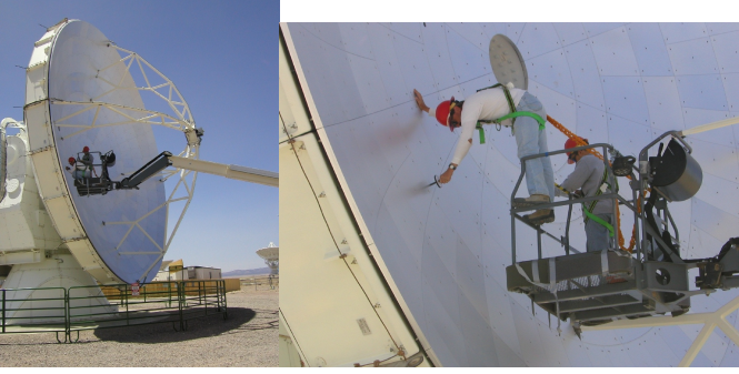
Fig. 9. Panel adjustment of the VertexRSI prototype antenna.
